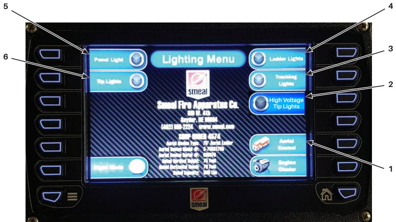
Figure 3-15. AL-11 Lighting Control Screen
